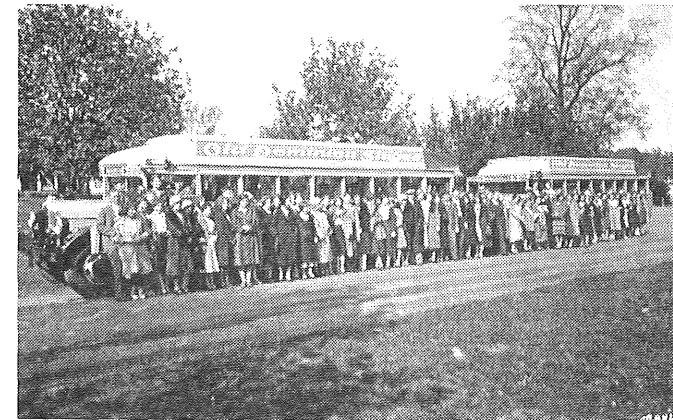
1930 Yellow Coach model 610, 33 passengers. Old Dominion Stages operated between Washington and Knoxville via Winchester and Bristol. Merged with Atlantic Greyhound during 1936 although Atlantic Greyhound had provided service for Old Dominion since 1932.
